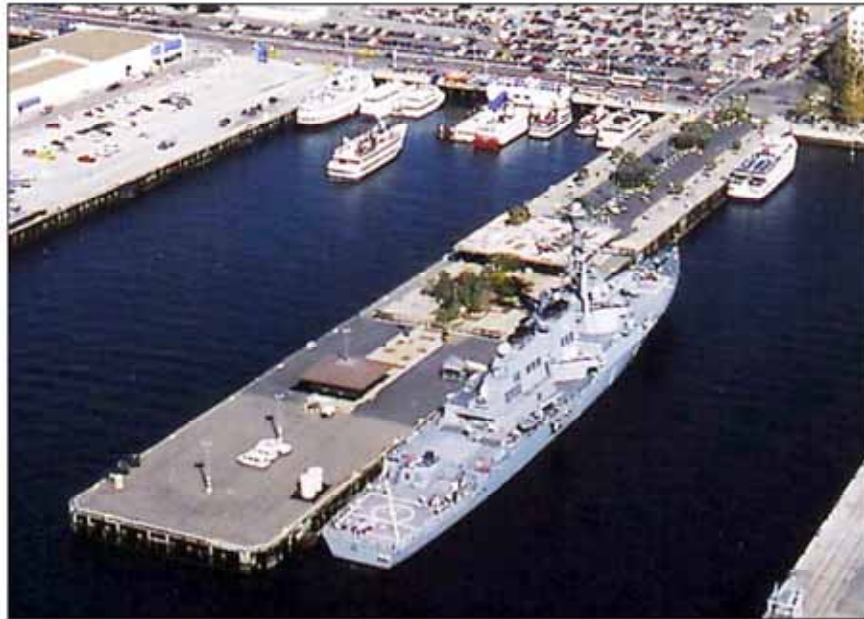
Existing Broadway Pier December 2006
